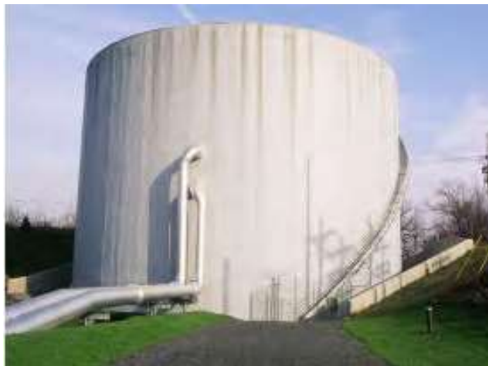
Figure 24: Cornell Chilled Water Storage Tank. Thermal storage tanks like this 4.4 M gallon storage tank on Cornell’s campus allow operators to shift periods in which chilled (or hot) water is generated, thereby shifting the timing of electrical usage for chillers (or heat pumps) used to generate the resource.
